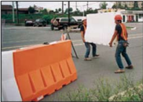
Figure 3. Empty Ballast-Filled Barrier Segments
