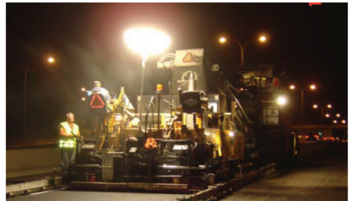
Figure 4 - Balloon Lighting in a Nighttime Work Zone
