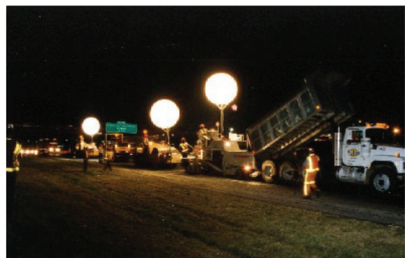
Figure 3 - Example of Balloon Lighting
