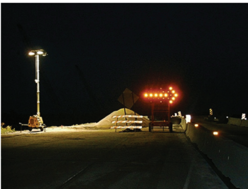
Figure 2 - Example of Portable Tower Lighting
