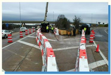
• Projects where the travel lanes are narrow and the speed is low, thereby reducing the possible angle of impact and the resulting deflection.
