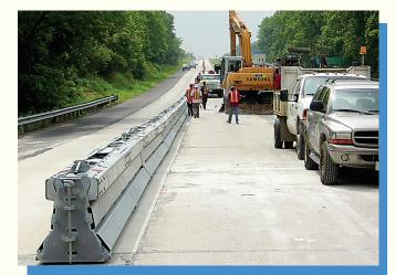
• Lateral displacement is usually in the range of 6 to 8 feet when impacted by a full-size pick-up truck. They can be anchored down to minimize deflection.
