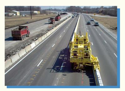
productivity within the work shift because setup time is minimized. Further, both workers and motorists are protected during the barrier move.
